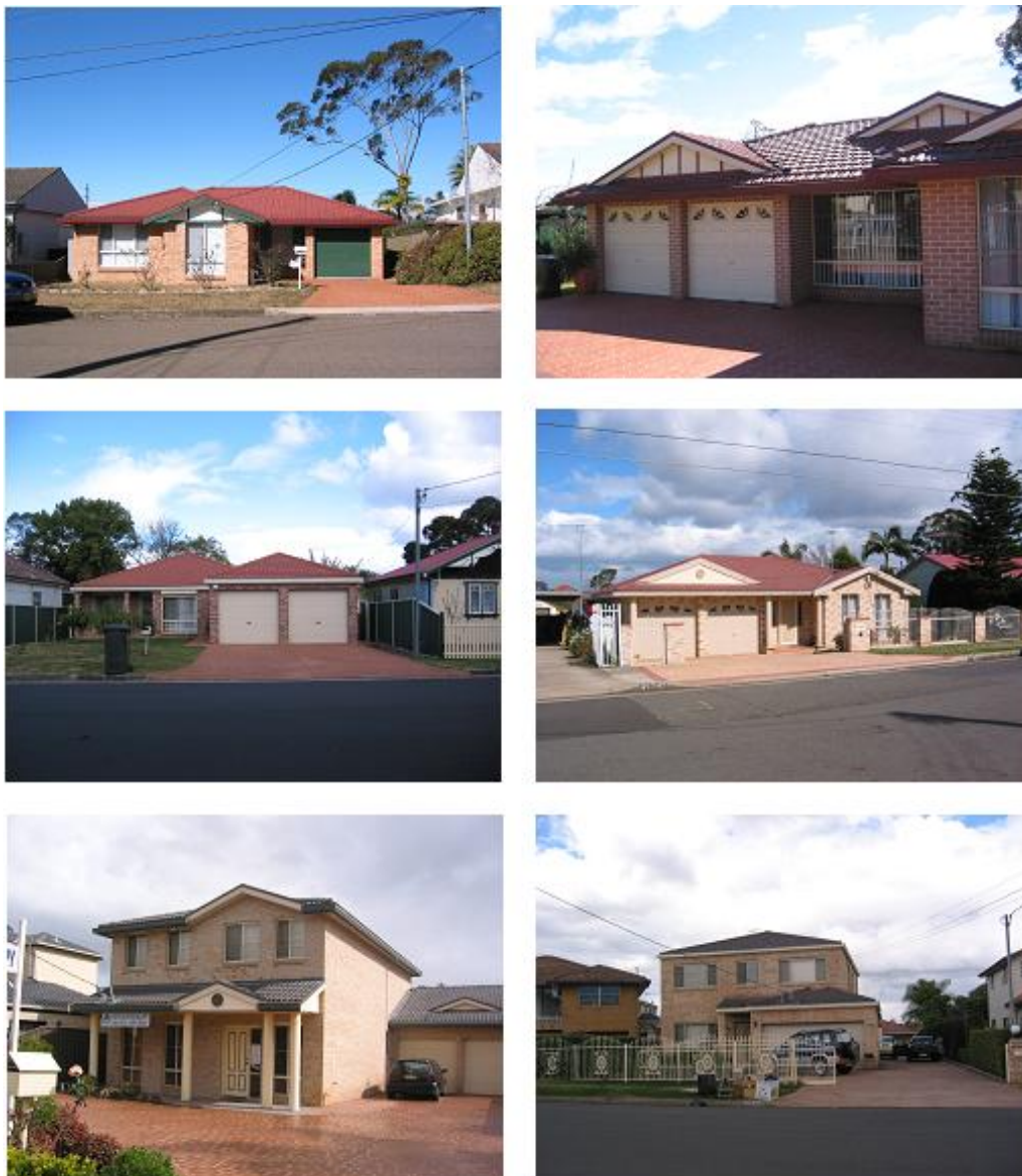
Figure 5. Typical installations in Sydney suburbs.
