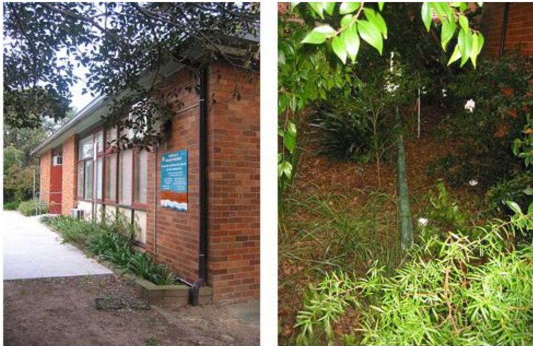
Figure 4. Storage gutter serving pipes to toilet cisterns in a community centre retrofit.
