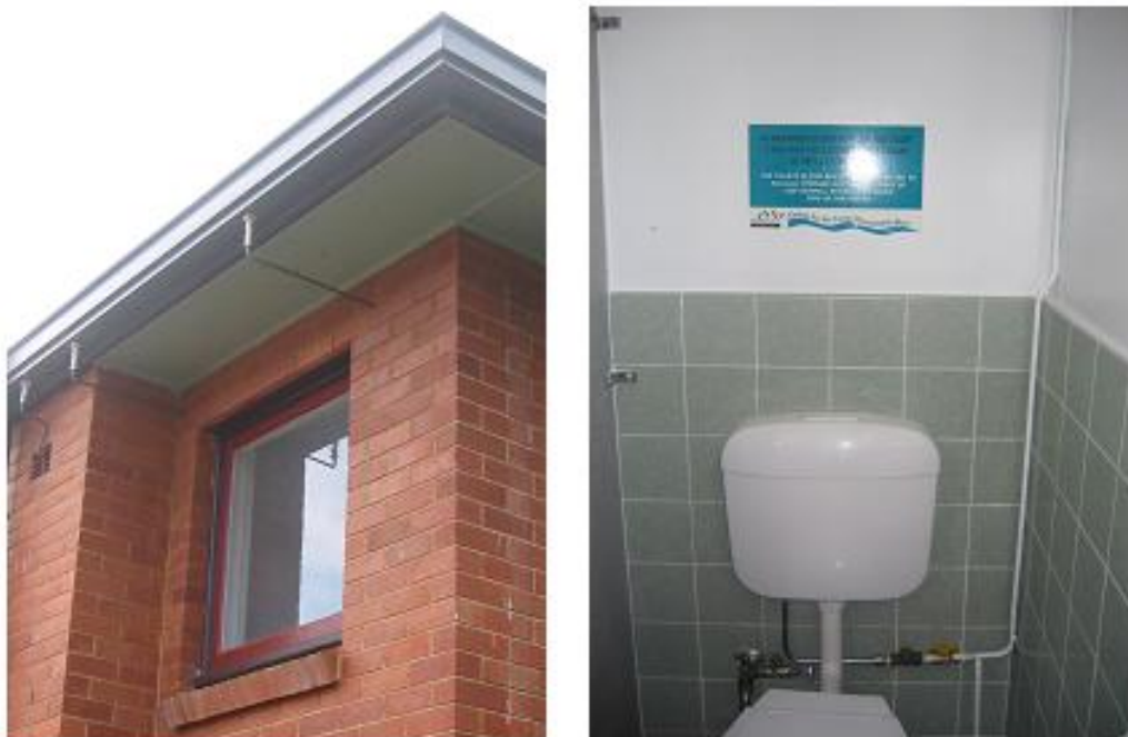
Figure 4. Storage gutter serving pipes to toilet cisterns in a community centre retrofit.
